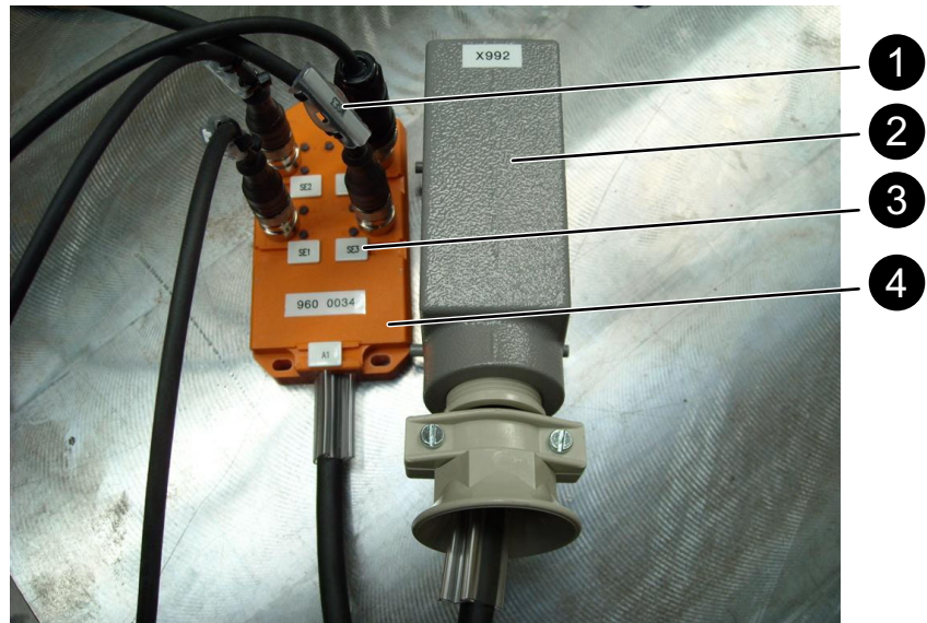
Fig. 4-42 Labelling of distributor and cables (illustration as an example)
